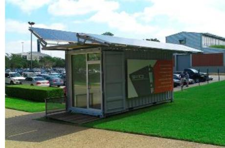
**GRID-CONNECTED SOLAR AND STORAGE:** [Florida's SunSmart Emergency Shelter](#) program equipped more than 100 public schools with solar + storage microgrid systems that can power lighting and electrical outlets at the schools if the grid is disrupted by a storm. Each school can provide emergency shelter for 100 – 500 people. During normal operations, the schools are able to use the solar panels to offset daily electricity usage and save \$1,500 - \$1,600 annually.
